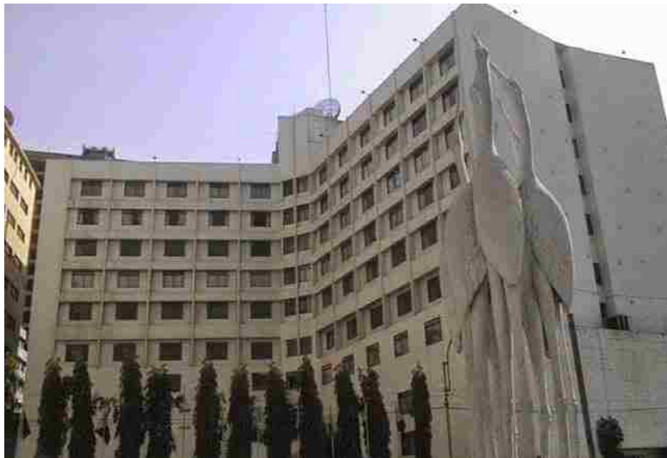
fig 29: Hotel Purbani, located in the Motijheel CBD area in Dhaka
