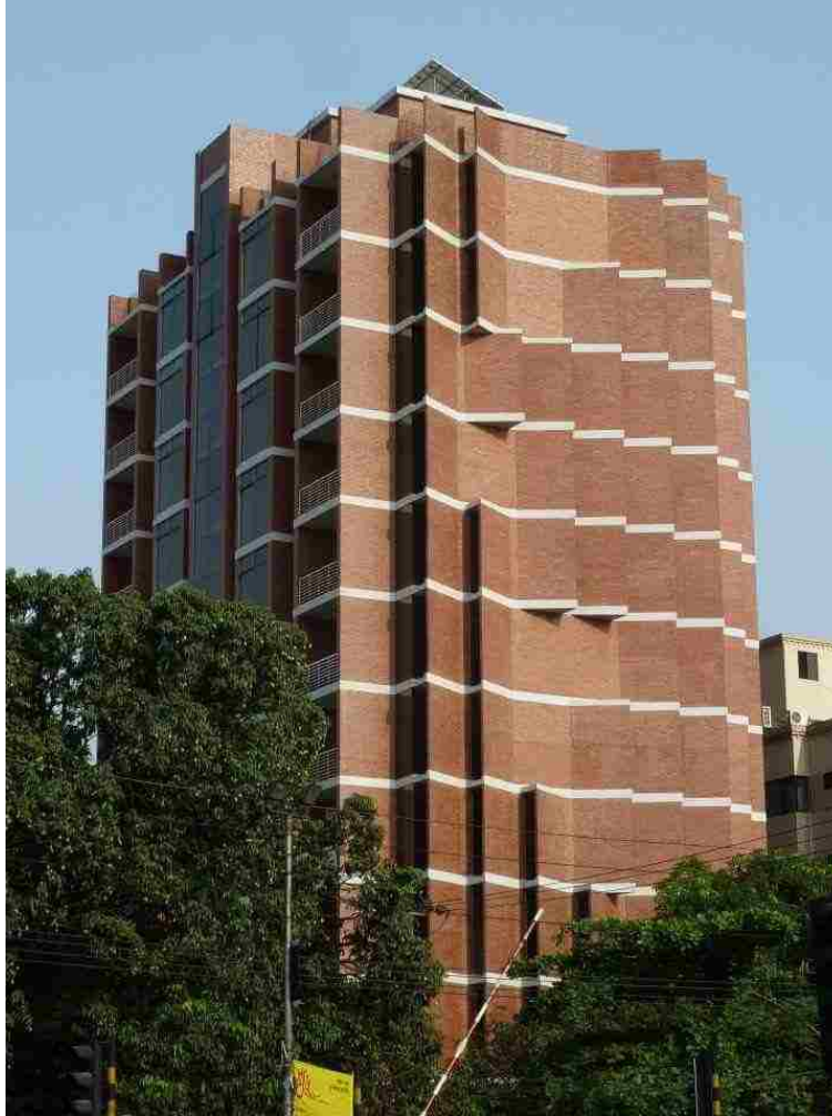
Figure 39: Using vertical fins for passive ventilation in warmer months of the year in Dhaka Bangladesh
