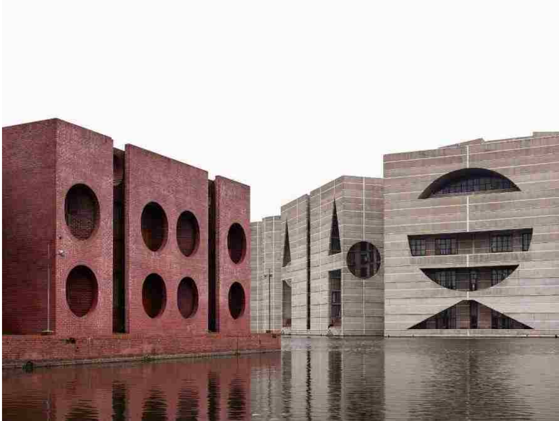
Figure 38: the parliament members' club with passive means of ventilation in red brick constructions
